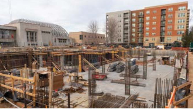
Construction of the Freyer — Newman Center
